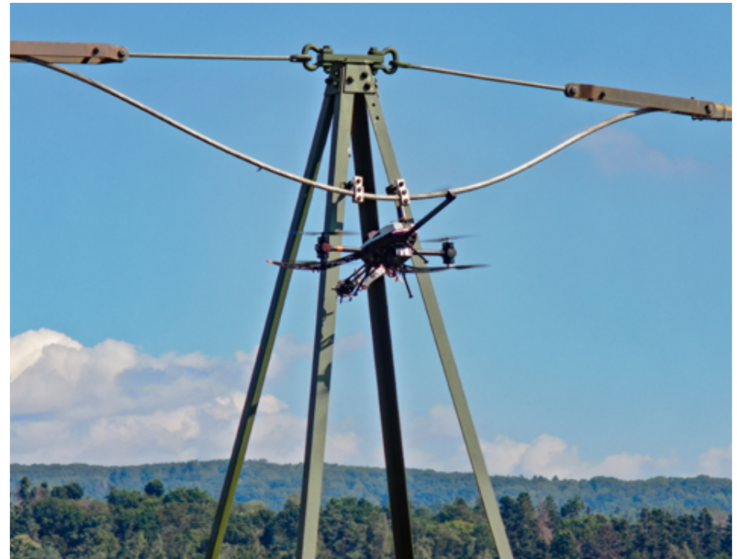
Corrosion analyses with drones are faster, standardised and safer
